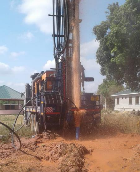
Well drilling September 2018
