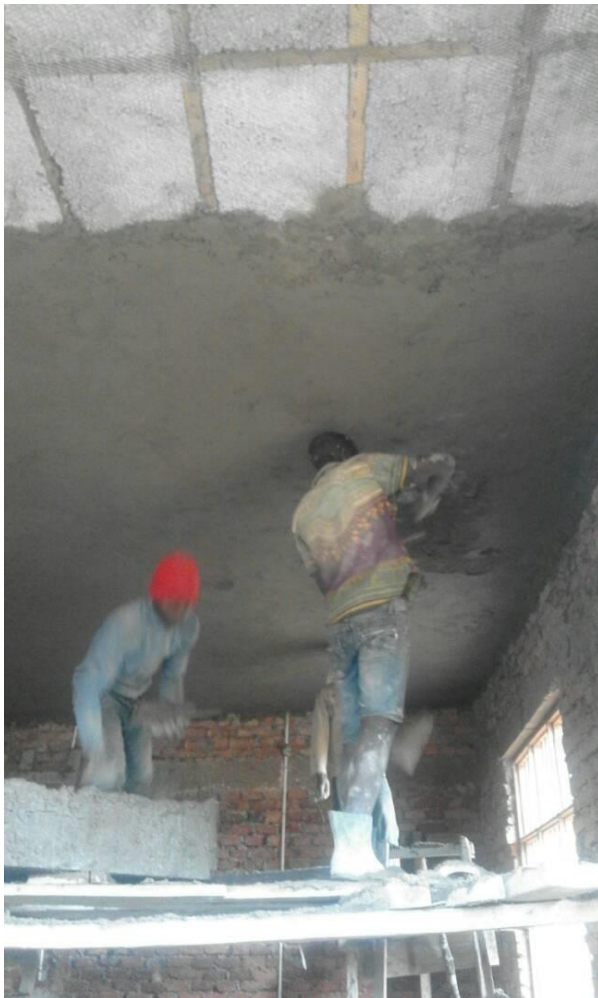
Plastering: photo taken 18.07.2018
