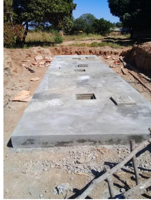
Waste water handling with a three-chamber system (under construction and ready)
