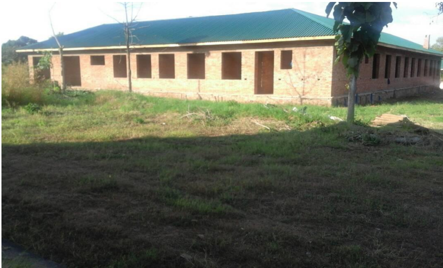
Building Photo taken in May 2018
