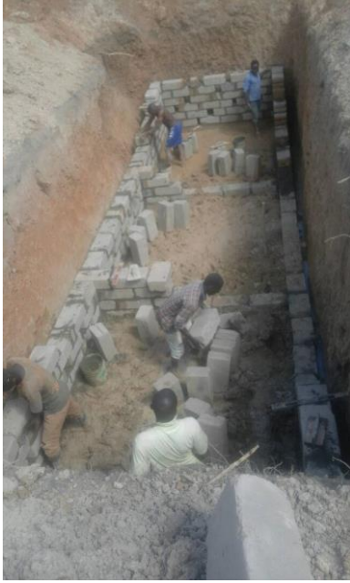
Waste water handling with a three-chamber system (under construction and ready)
